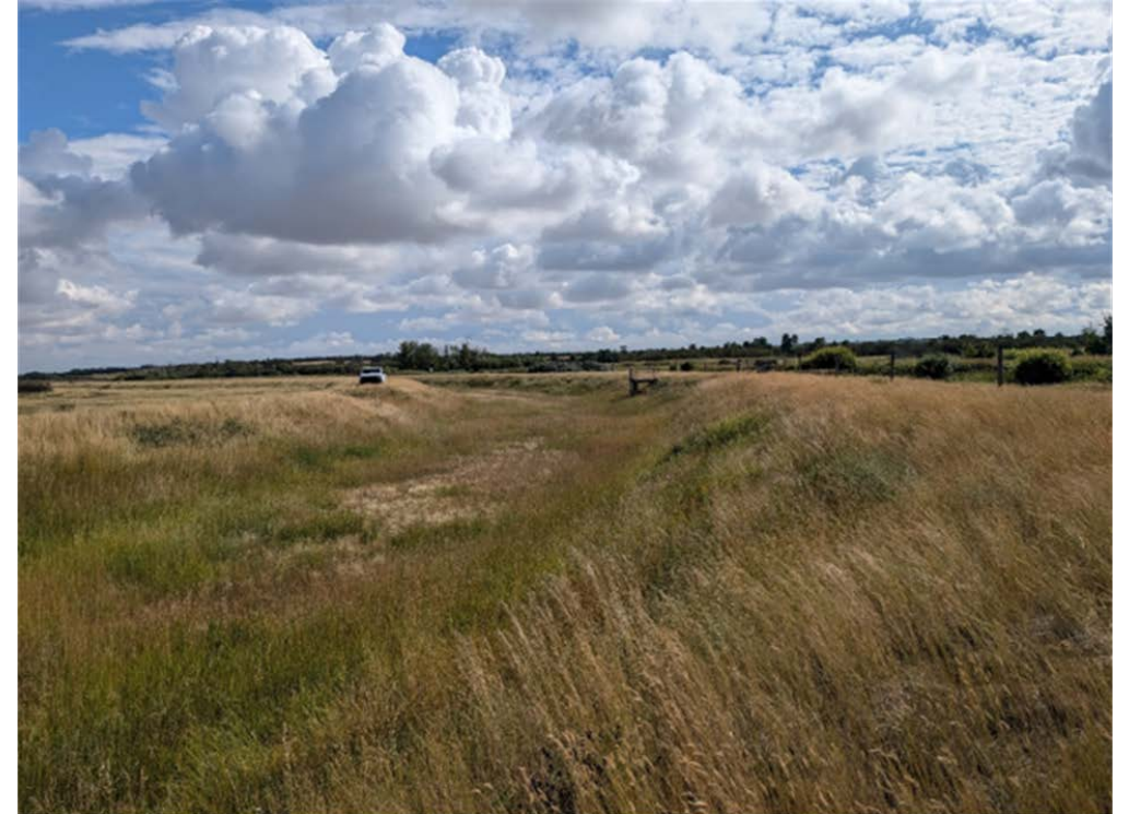
Photo of existing dry Westside Main Canal
