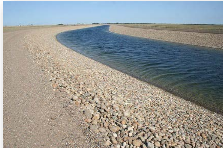
Eastside Canal (28 m 3 /s)
