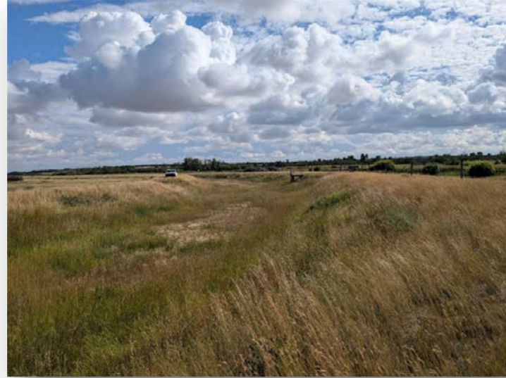
Existing Dry Westside Main Canal
