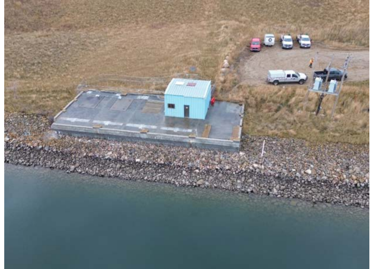
Photo of the existing Westside Pump Station
