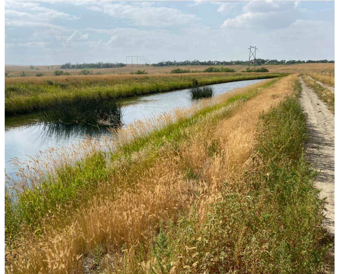
Photo of the existing wet (in use) Westside Main Canal
