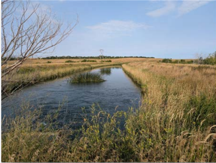
Existing Wet Westside Main Canal
