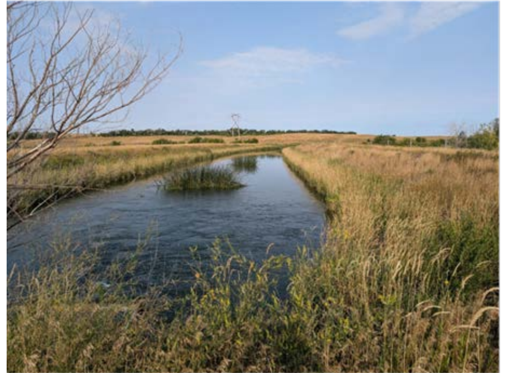
Photo of the existing wet (in use) Westside Main Canal
